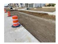
4. GM and Engineer responded to reports of drainage issues on Angus Drive. Loutfall areas need to be graded so the area will drain properly. Trash collection and silt fence removal is also needed in this area.
